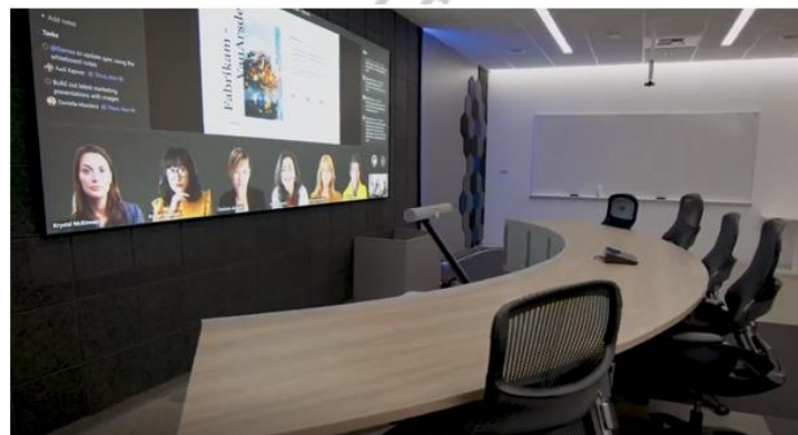
Microsoft's new main room shown at The Hive, with 21:9 Front Row projection screen, floor mounted projector with VC soundbar mounting arm.
